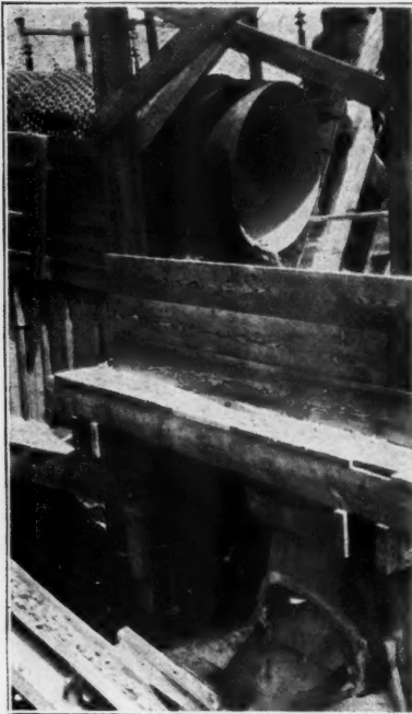
Discharge End of Scalper
